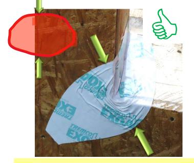
I prefer the "Football" because the overall width at the inside corner is substantial. There will be a little wrinkling, but as long as the membrane is properly rolled, and do not extend to the edges, the detail works well.
