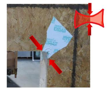
The "Bow Tie" is thinner at the middle, which is where the coverage must happen for this detail to work successfully. It is easy for the installer to mistakenly make the middle too thin or stretch the membrane and therefore, the inside corner might not have proper coverage of the membrane.
